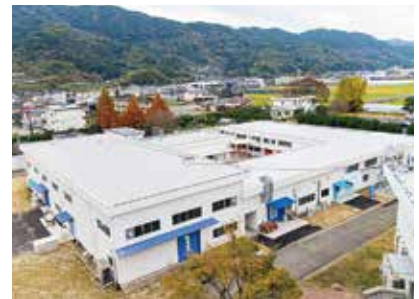
実験・実習棟 Building for Technical Applications and Experiments
