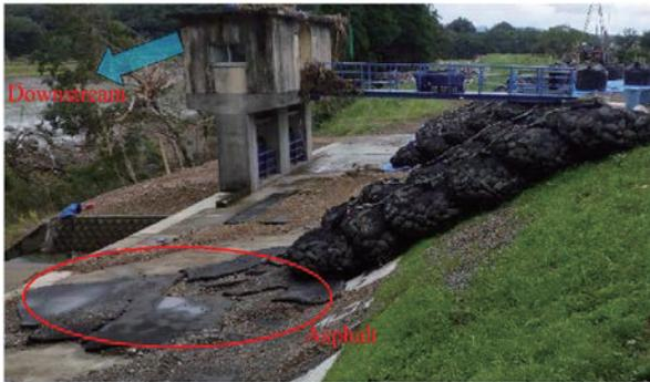
Fig. 8 Outflow asphalt pavement of L55k
