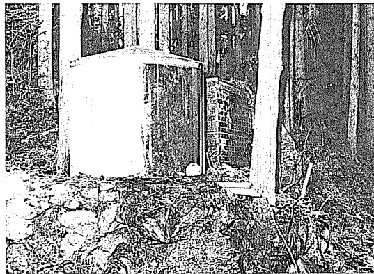
Fig. 51 The water tower at Arahira
